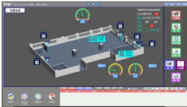
Air Conditioning Control
